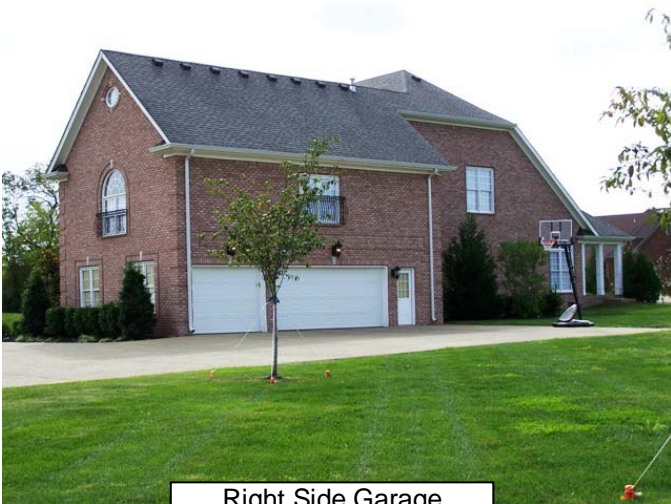
Right Side Garage
